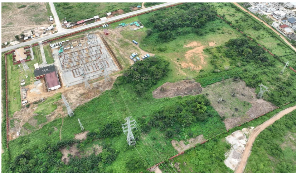
Figure 1: Aerial view of Bingerville substation, looking south (campaign Dec. 2023)
