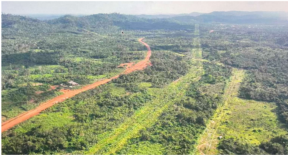
Figure 2: Access to the proposed Dunkwa II Substation
